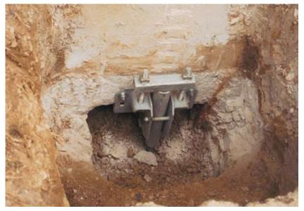
Completed helical pile and bracket
