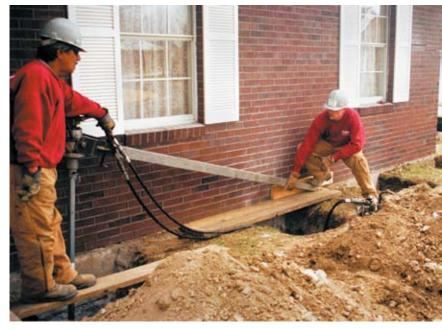
Helical pile installation by hydraulic driver
