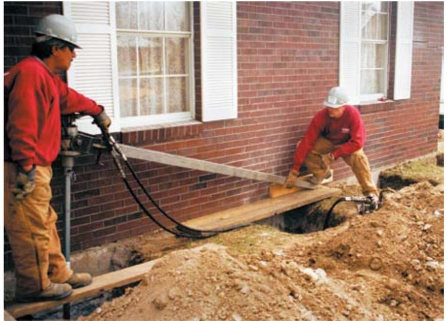
Helical pile installation by hydraulic driver
