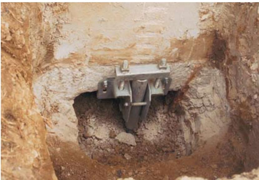
Completed helical pile and bracket
